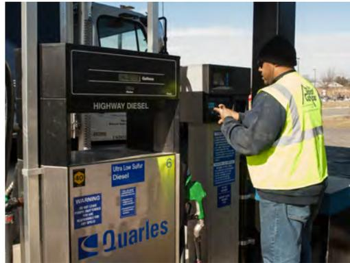
*The OPW FSC3000™ Fuel Site Controller inside the C/OPT™ Fuel Island Terminal can track and report fueling transactions by driver and/or vehicle.*
